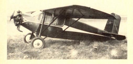
which had been faired with sheet metal -by streamlined tubing. Another was replacement of the rubber-ring shock absorber system by an oleopneumatic type that incorporated a long compression strut, running from the axle to the point where the front spar of the wing attached to the fuselage. ATC 321 was awarded to the Model E in May 1930.
